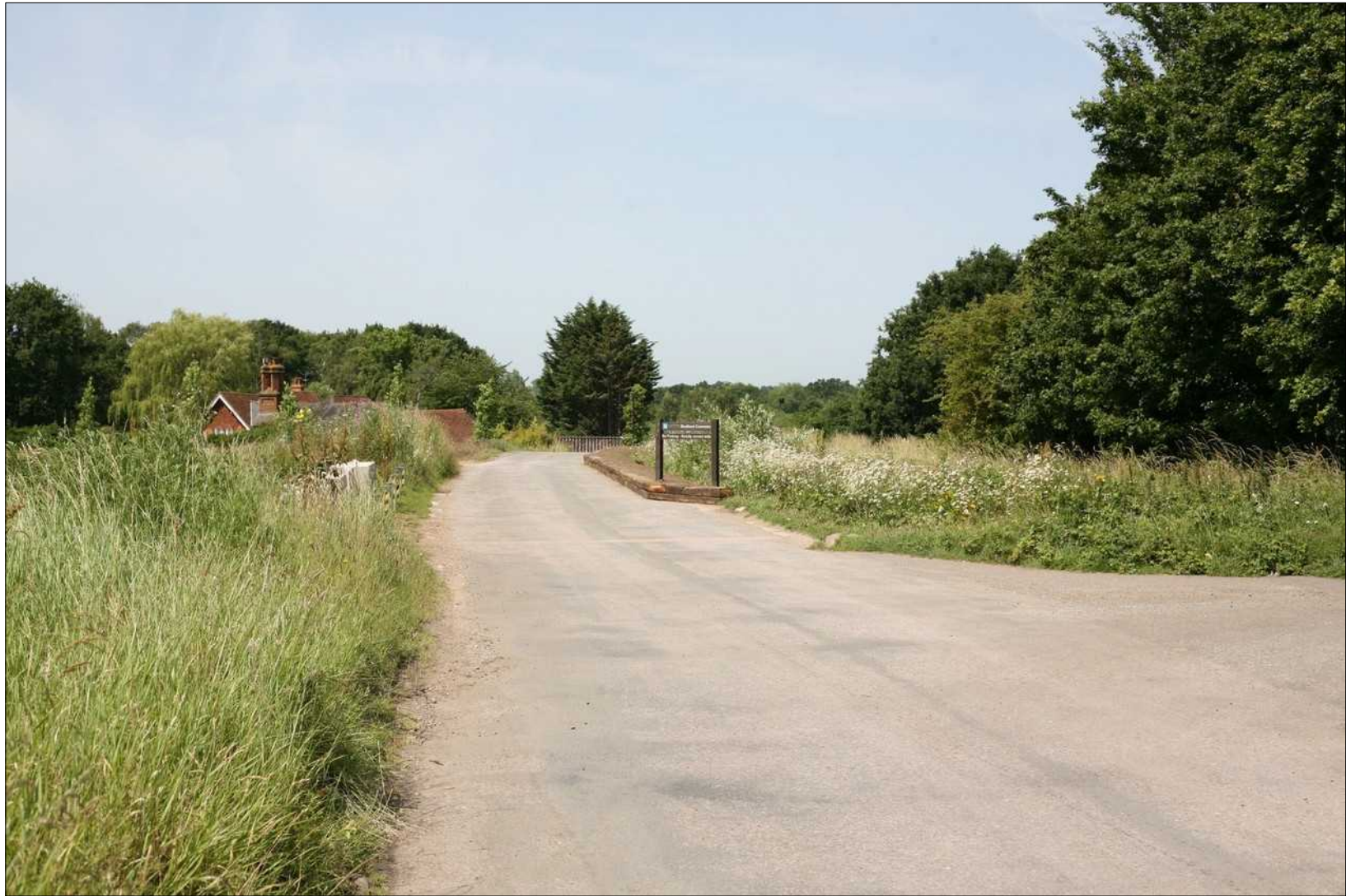
Dagley Lane looking from Horsham Road
