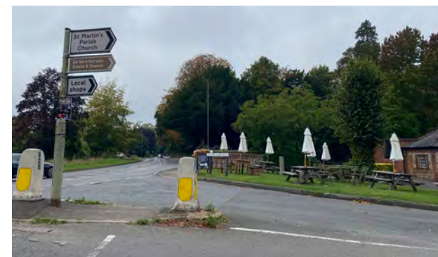
Figure 41. Ockham Road junction with Epsom Road proposals include junction tightening, introduction of raised table and parallel crossing.
