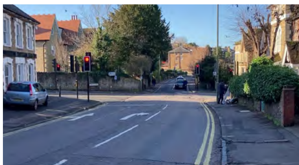
Figure 28. Removal of short right turn lane at Waterden Road junction will offer space for dedicated (mandatory) eastbound cycle lane (uphill), and provision of signal-controlled crossing on the eastern arm.
