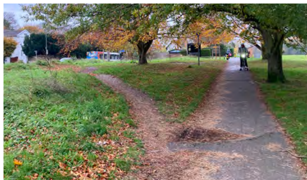
Figure 75. Shalford Park shared use path requires widening and resurfacing, as in many locations tree roots have damaged the surface. Existing desire lines to Pilgrims Way bus stop to be formalised.
