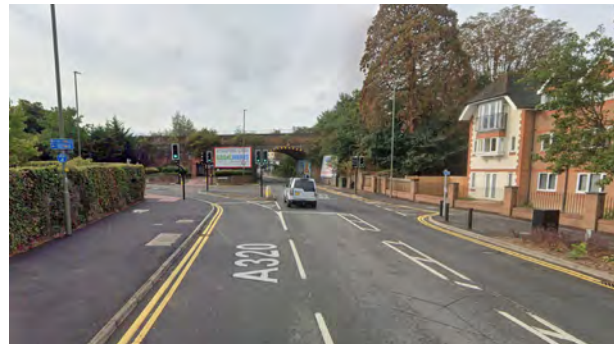
Figure 15. Stoke Road / Nightingale Road junction: There is no crossing on the north arm of the junction to allow access to the shared use path. Source: Google Street View.
