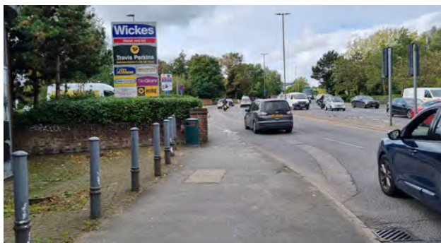
Figure 21. Existing shared use paths on the A25 have inconsistent width and at locations are very narrow. Improvements to the facilities are required to enhance the connectivity of the network.
