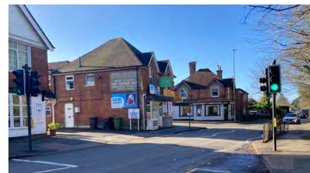
Figure 30. Existing signal-controlled crossing near High Path Road to be upgraded to toucan and the guardrail removed.
