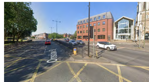
Figure 14. Onslow Street: dual carriageway with high traffic flows. Existing footways have guardrail. Opportunity to widen the footways to accommodate shared use path to provide access to the town centre. Source: Google Street View.
