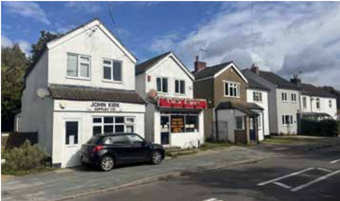
Guildford Road - residential converted for business uses
