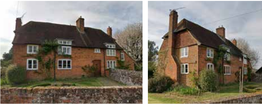
Grade II Listed West Wyke Farm as seen from Pound Farm Lane (Google)
