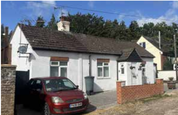
Pinewood Road - painted render with brick lintels
