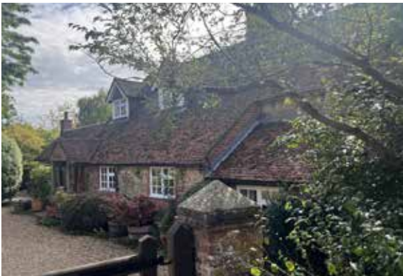
Harpers Road – York House, Grade II Listed
