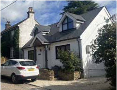
Pinewood Road - pitched roof dormers
