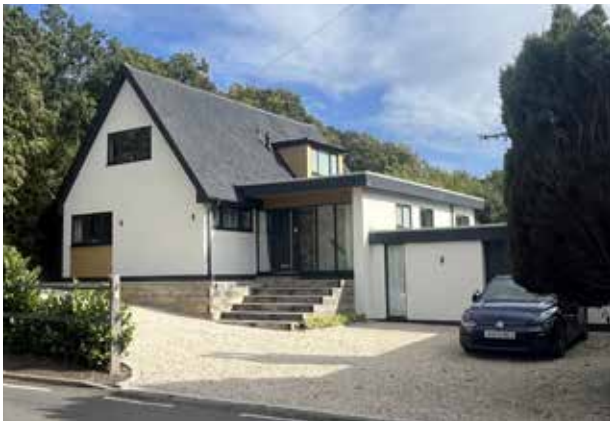
Ash Hill Road - contemporary remodelling
