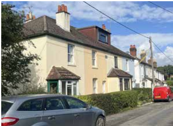
Harpers Road – tiled porches, sash windows & chimneys
