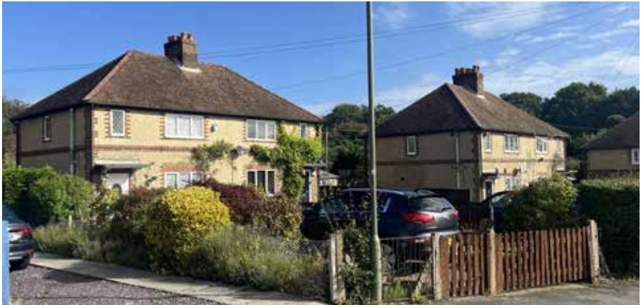
Wyke Avenue – natural render with red brick bands, quoins window surrounds and lintels
