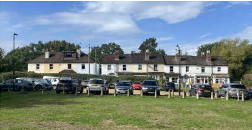
Harpers Road – Short terraces with varied colours overlooking parking yard
