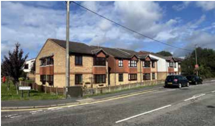
Guildford Road - 2 storey apartments
