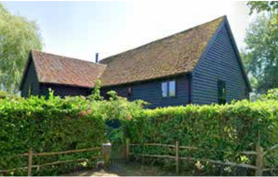
Grade II Listed The Oak Barn (Google)
