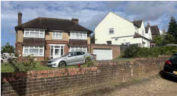
Ash Hill Road - brick corbels and quoins to front door surround
