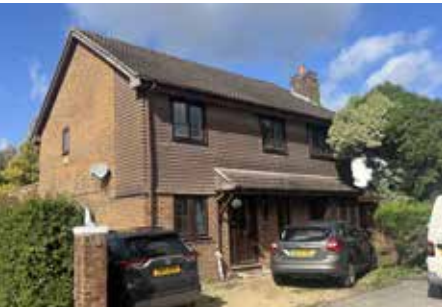
Pinewood Road - brown brick & tile hanging
