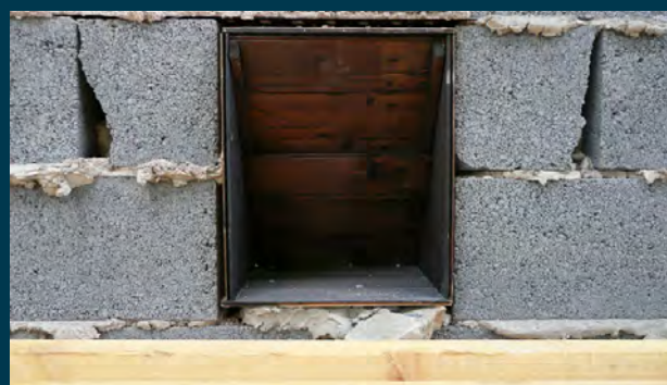
Hopper providing sheltered fly-in access (see Schofield, 2008).
