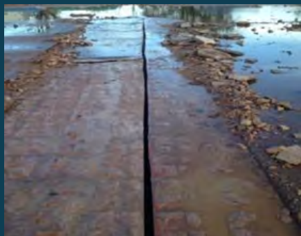
Diamond cut through culvert slab
