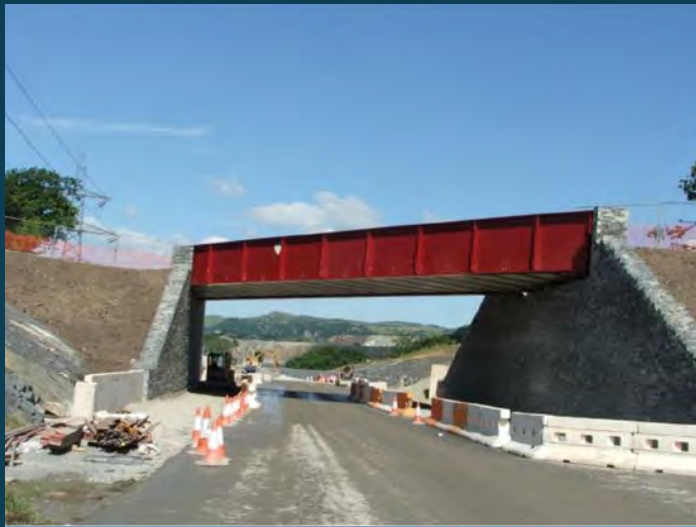
Bridge crossing during construction
