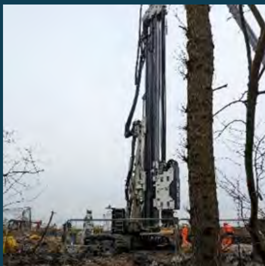
Noise measurement of Auger piling
