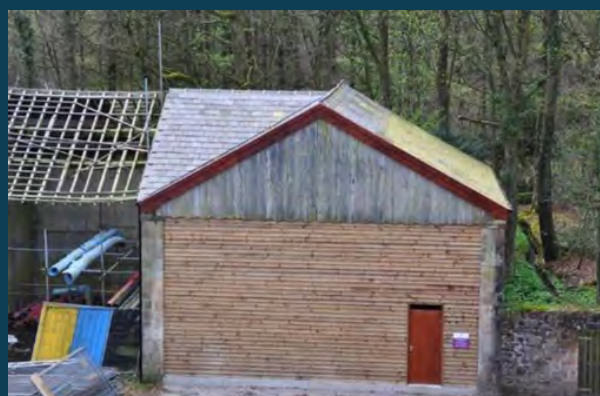
Detail of the compensation building (bat barn)
