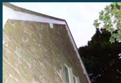
Bat access point at gable apex
