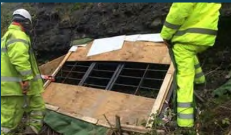
Partial closure of the adit entrance
