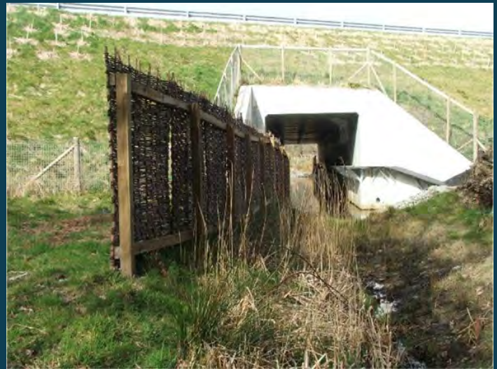
Culvert with hurdle fencing guide
