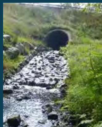
The culvert with stream flowing through
