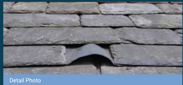
Bat access point at gable apex
