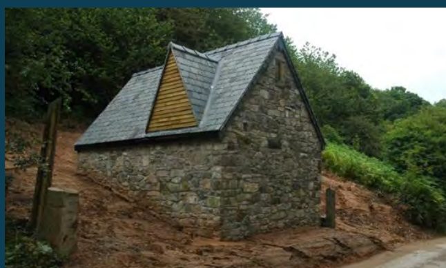
Replacement roost July 2011 (south-western elevation)
