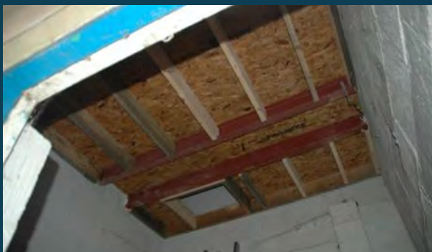
Internal – ceiling inserted 1.5 m below flat roof
