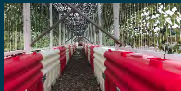
Interior of semi-permanent scaffolded flightline
