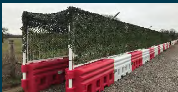
Semi-permanent scaffolded flightline
