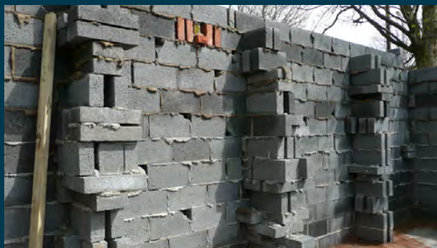
Cavity wall comprising compressed cinder block inner wall with brick outer leaf. Walls deliberately left rough for additional perching/roosting and with deep wall cavities also.
