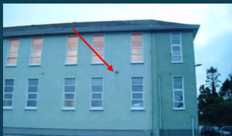
Ventilation grille used by soprano pipistrelles
