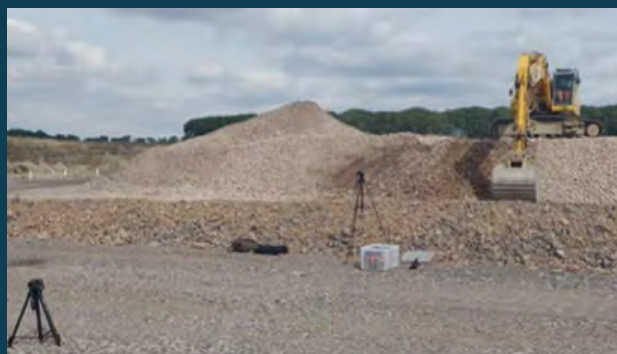
Noise measurement of stockpile management
