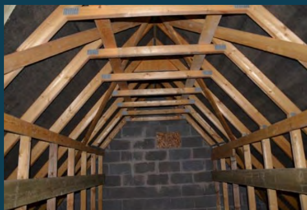
A modified open-plan trussed roof was used with a rough timber ridge board inserted at the apex and an additional false purlin inserted 600 mm above floor level
