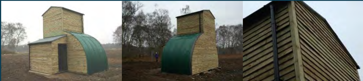
Completed conversion – 2009. Timber wedges (right) were added to create gaps behind the timber cladding
