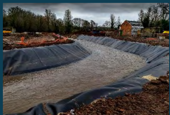
Diversion of river in place
