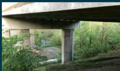
View of PNV Viaduct, looking east.
