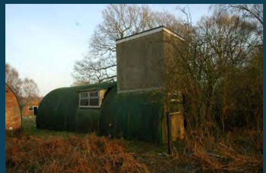
Building prior to start of works
