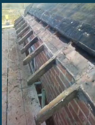
Stripped wall plate
