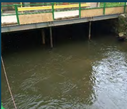
Western end of culvert
