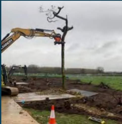
The monolith is lifted into position
