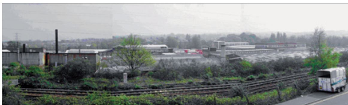
Figure 7: View over the estate from Midleton Industrial Estate
